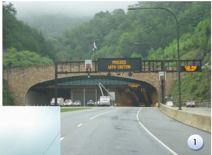
1. Corridor F: US 25E Cumberland Gap Tunnel
